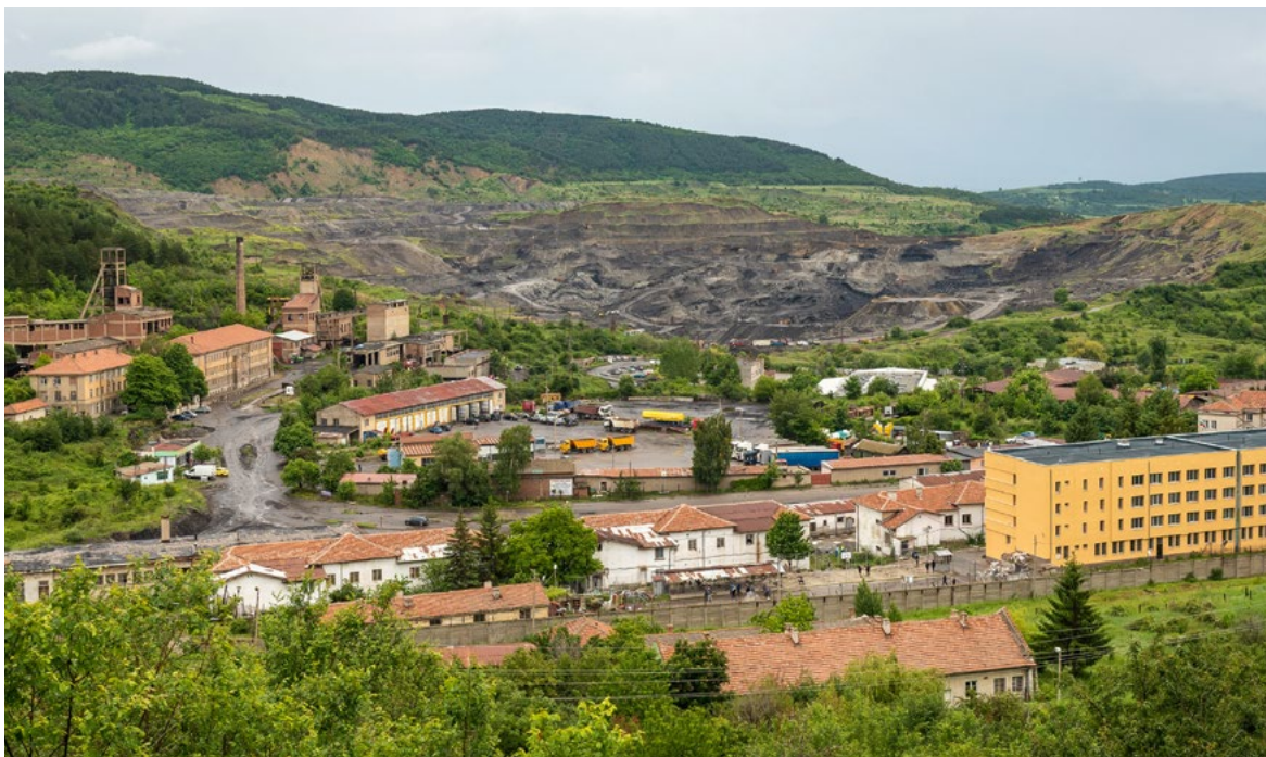
One of the last operating surface mines in Bobov dol along with its supporting infrastructure.
