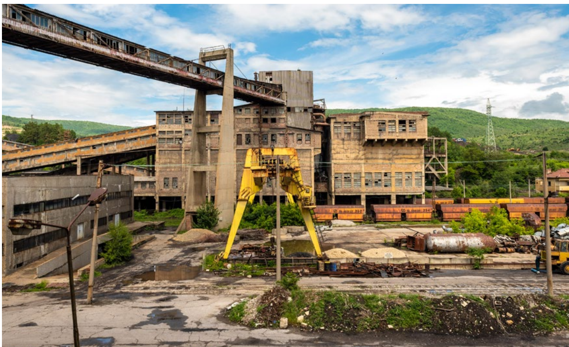
The enrichment factory is still operating albeit at low capacity. It was built around 1944 next to the underground mine Babino which closed at the end of 2016.
