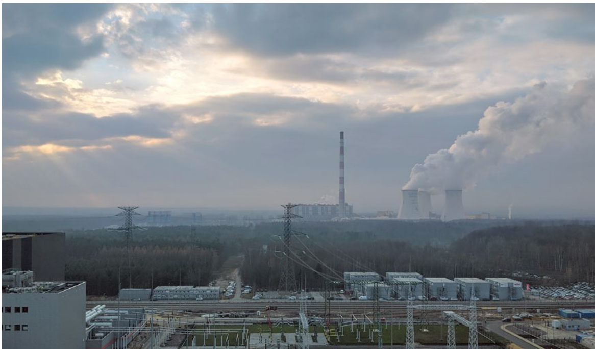
Jaworzno power plant is one of the biggest coal-fired thermal power plants in Poland with installed capacity of 1 535 MW. Poland's energy sector is heavily reliant on coal with a 78% share in 2018.
